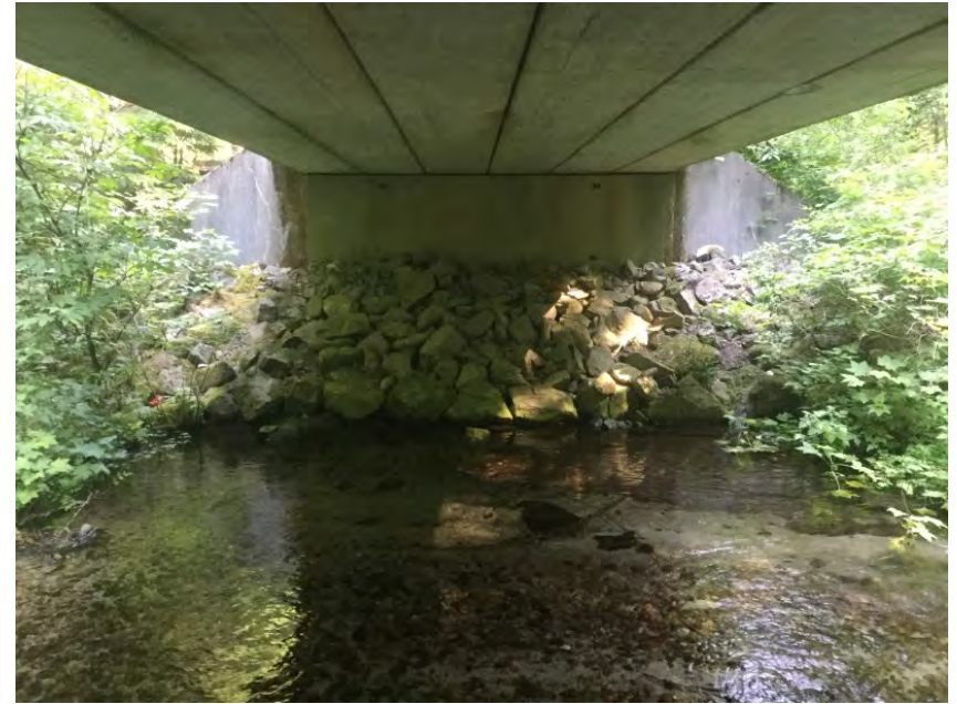
Left Bank Abutment when facing downstream
