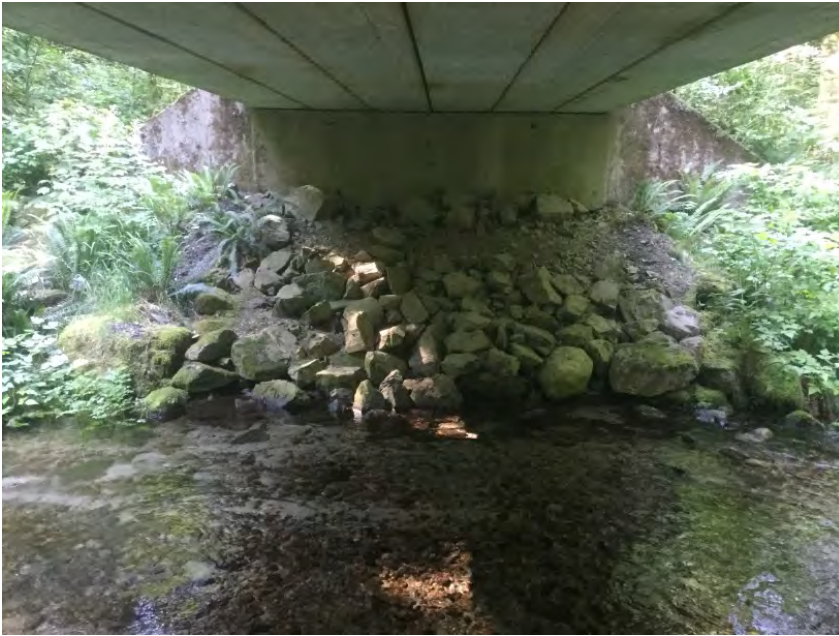
Left Bank Abutment when facing downstream
